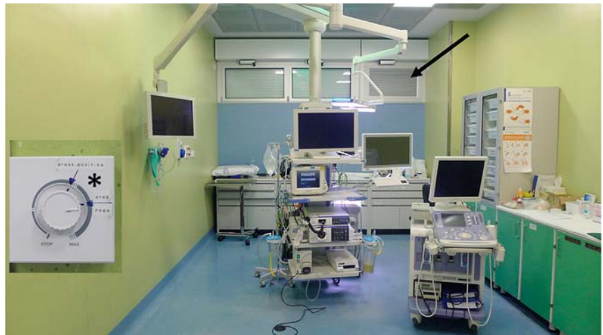
► Fig. 2 Endoscopy room with a dedicated ventilation system (black arrow) to guarantee a negative pressure (asterisk).
