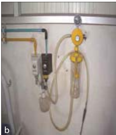
Figure 2b: Photograph showing the wall suction apparatus used for vacuum application
