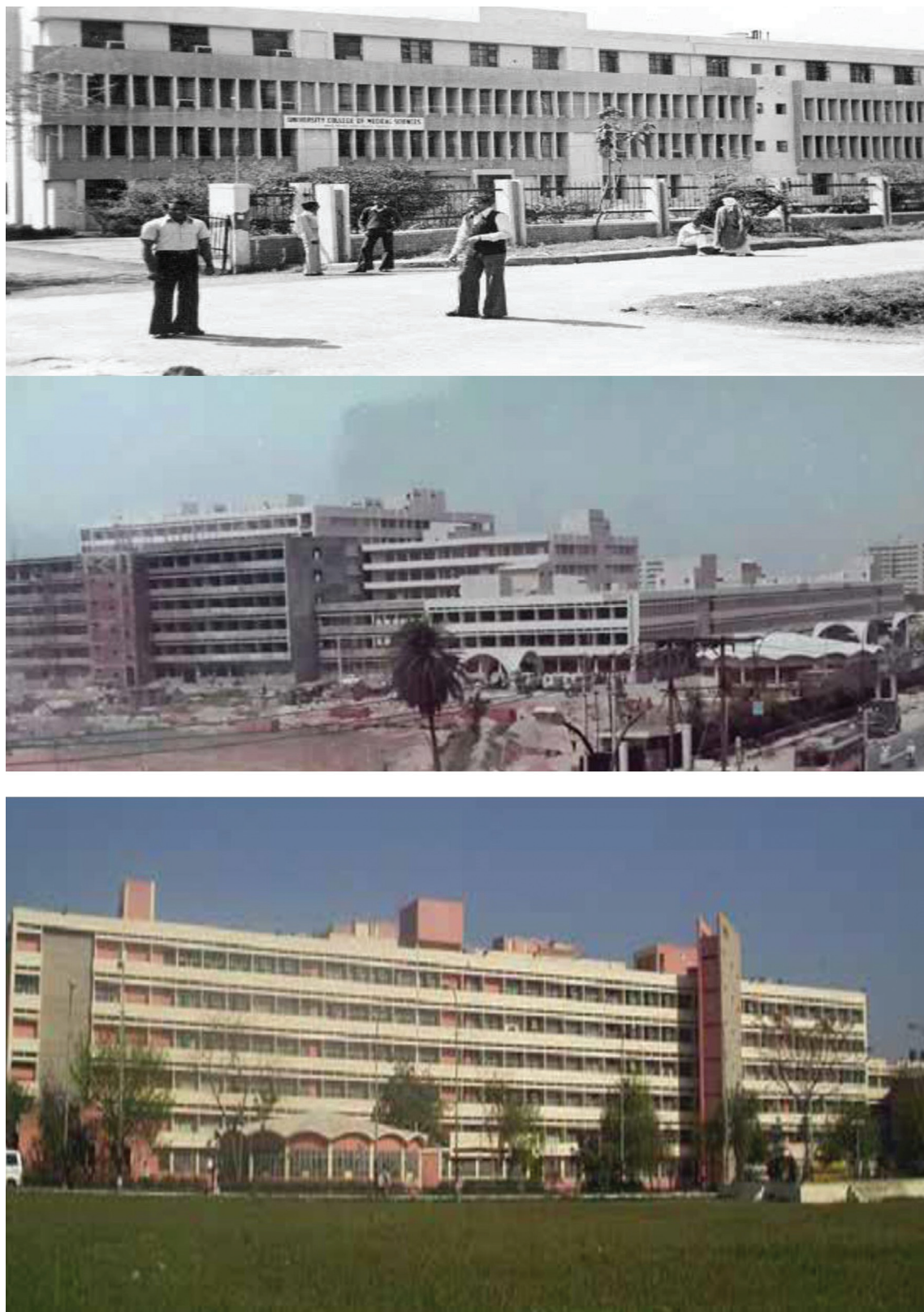
Fig. 1 (topmost): UCMS Building at Safdarjung Hospital (1973); (middle): Formation of UCMS (1985–87); (bottom): UCMS (2020–21).
